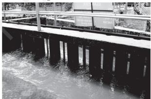
Fig. 18.4 Grit and sand removal tank
