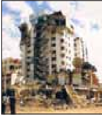
Fig. 3.3a: Destruction caused by an Earthquake in Gujarat
