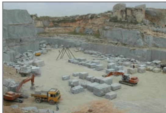
Fig. 3.7: Quarrying of limestone
