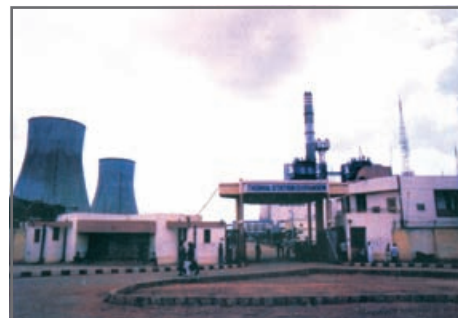
Fig 3.12: A view of a Thermal Power Station
