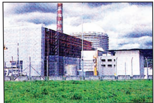
Fig. 3.18 : Nuclear power station , Kalpakkam
