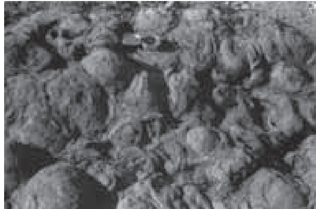
Fig.6.4 : Exfoliation (Flaking) and granular disintegration
