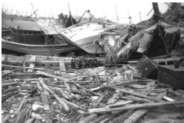
Figure 7.3 : Tsunami Affected Area
