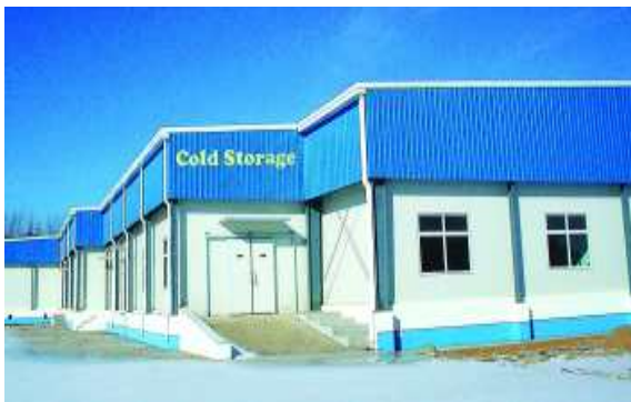
Fig-22 Cold storage unit
