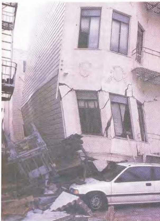
An earthquake can damage buildings
