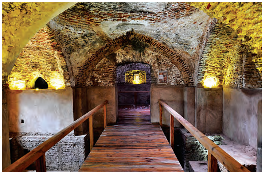
Picture 2. Inside the beautiful Shahi Hamaam after repair.
