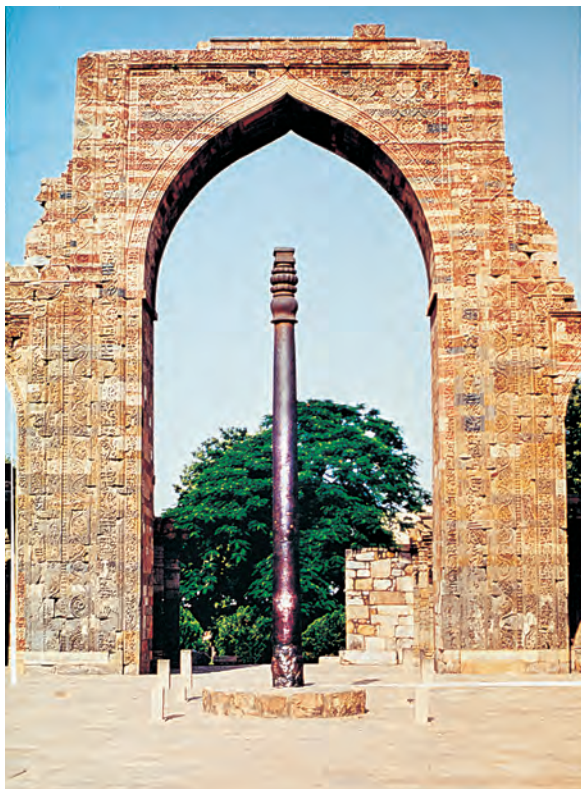
The iron pillar at Mehrauli.
