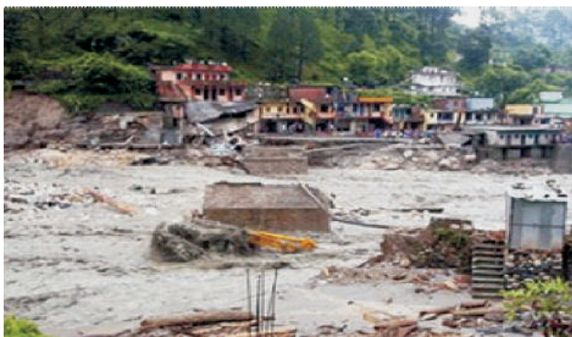
Devastation due to flash floods in Uttarakhand
