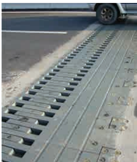
Figure 8.3 Expansion joints for safety
