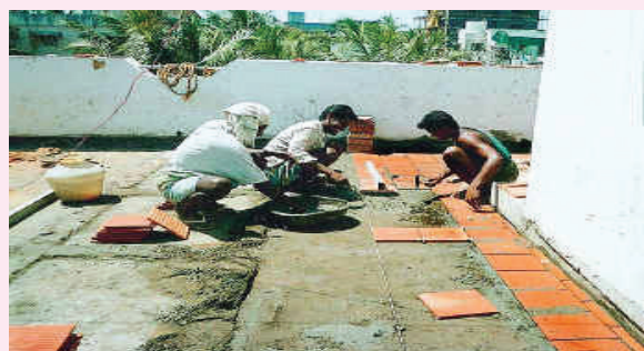
Mason fixing the tiles on the floor.
