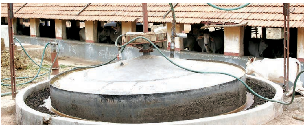
Fig.3.11-Biogas (Gobar gas) plant
