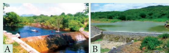
Figure 8.4: Constructions under TAP A. Check Dam B. Percolation pond
