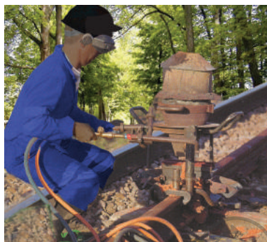
Figure 3.11 Thermit process for joining railway tracks
