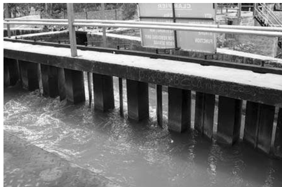
Fig. 18.4 Grit and sand removal tank
