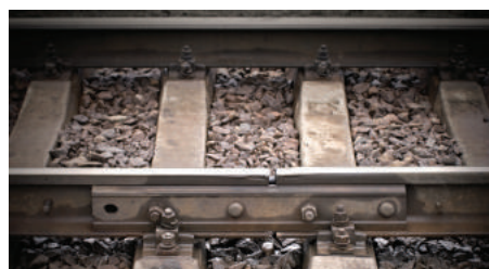
Figure 7.1 Gap in railway track
