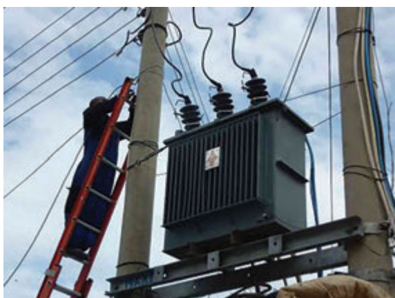
Figure 4.37(b) Roadside transformer
