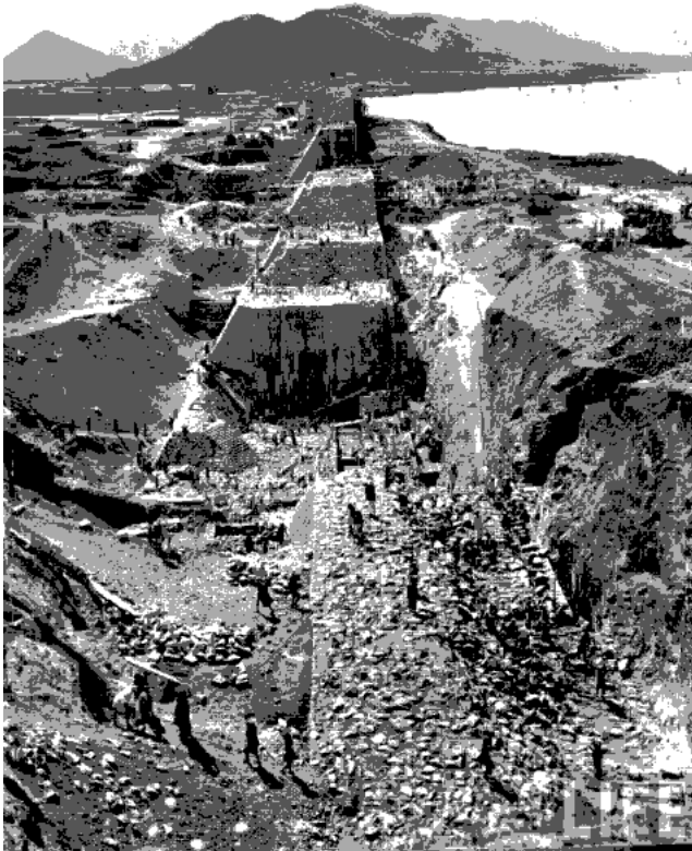
Fig 5.2 : Tungabhadra Dam Construction - 1952
