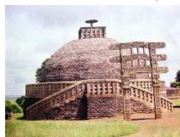
Fig: 20. 9 Sanchi stupa in Madhya Pradesh. It is one of the most important stupas built by King Ashoka. Can you identify the hemisphere, the platform, the umbrella and the fence?
