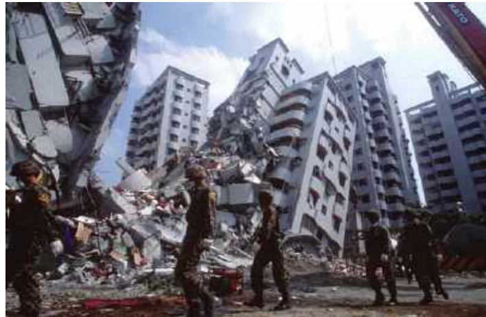
5.2: Scenes of destruction due to earthquake
