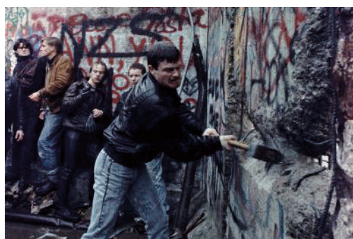
Demolition of Berlin wall
