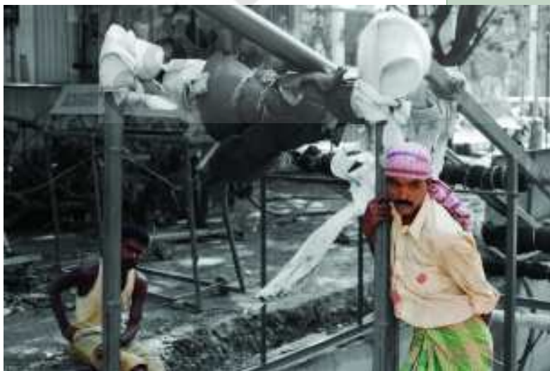
Fig 21.5 Road Laying Work
