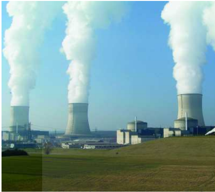
Fig 6.6 Nuclear Power Plant - Cattenom
