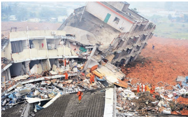
Effect of Earthquake
