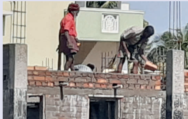
Mason packing bricks for constructing a wall between two pillars
