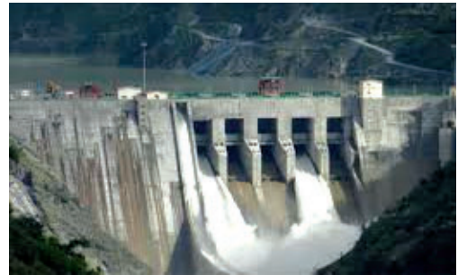
Baglihar Power Project
