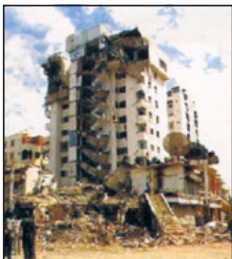
Fig. 3.3a: Destruction caused by an Earthquake in Gujarat
