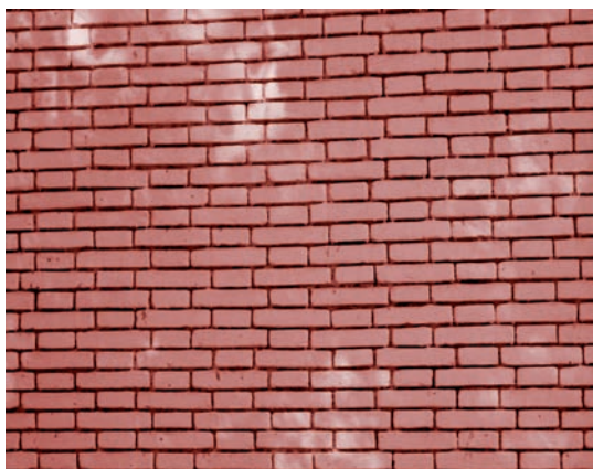
(a) Brick wall
