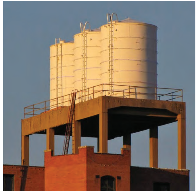
Overhead water tanks
