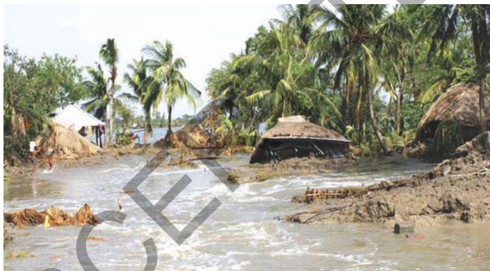
Fig 4.4 : Impact of Aila : (Top) broken embankment, (Bottom) repairing embankment
