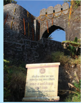
Figure 1.11 : Sinhagad Entrance Gate
