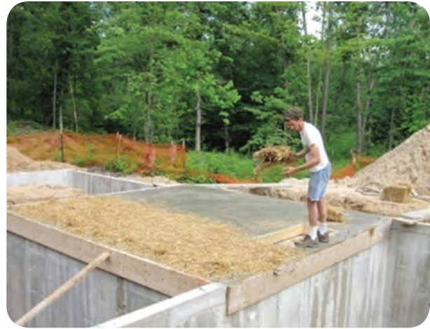
Covering the concrete with wet sand
