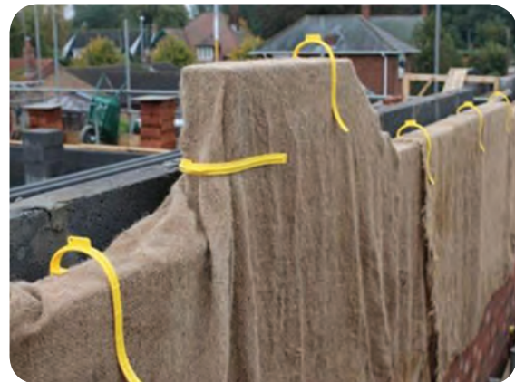
Covering the concrete with, jute bags
