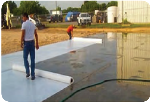
Covering concrete with polythene bags
