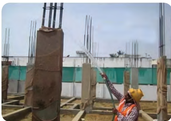
Cured by covering with wet sack
