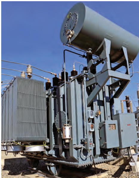
Fig 6.13 Protective Devices of Transformer
