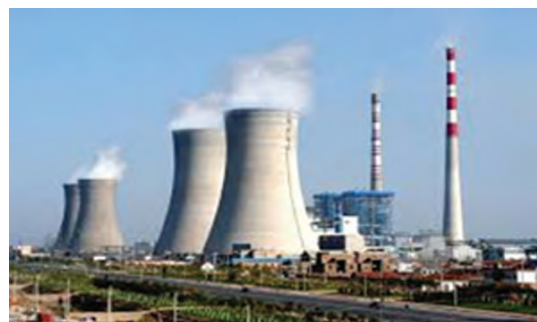
Thermal Power Plant (Neyveli)
