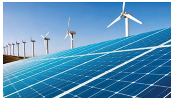
Solar and Wind Plant (Kamuthi)
