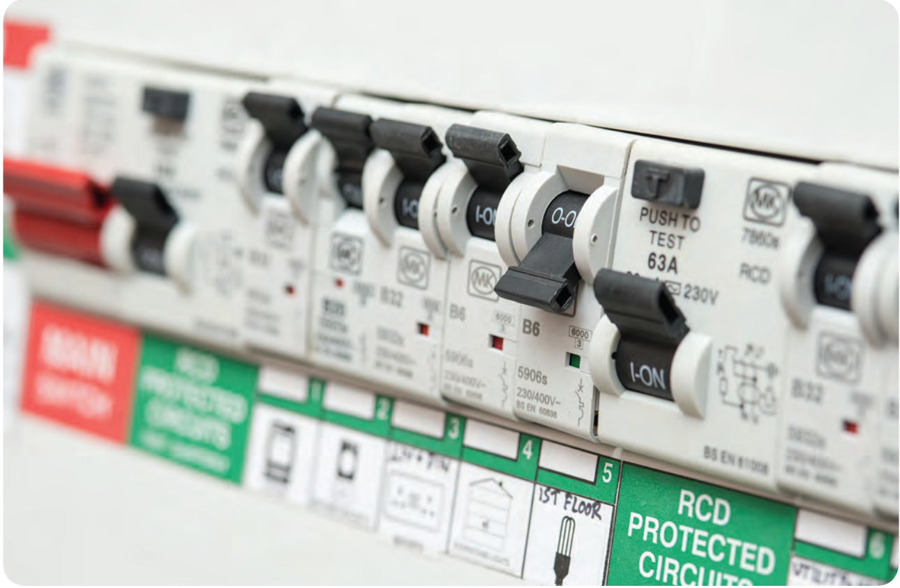
Wiring of the Distribution Board with RCD (Single Phase Consumer Unit) (From Energy Meter to the Main Distribution Board)
