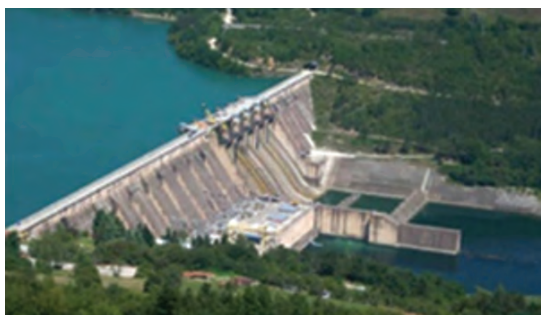
Hydro Power Plant (Mettur)
