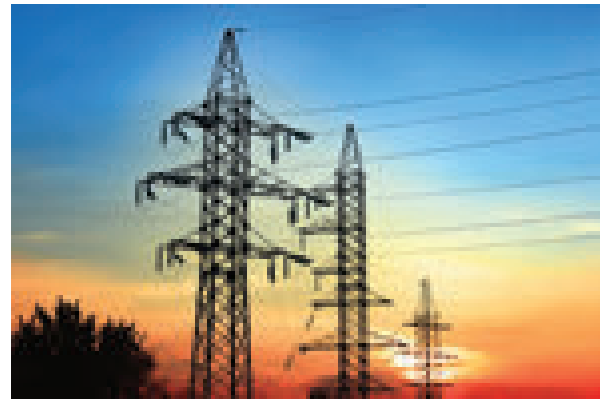
Fig. 1.7 Latticed steel tower
