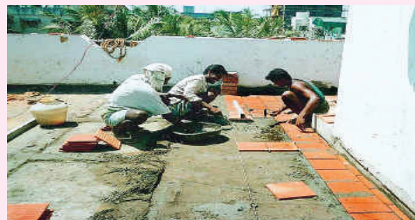
Mason fixing the tiles on the floor.
