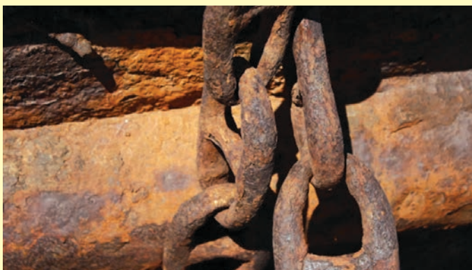
Fig 3.6. Rusting of iron
