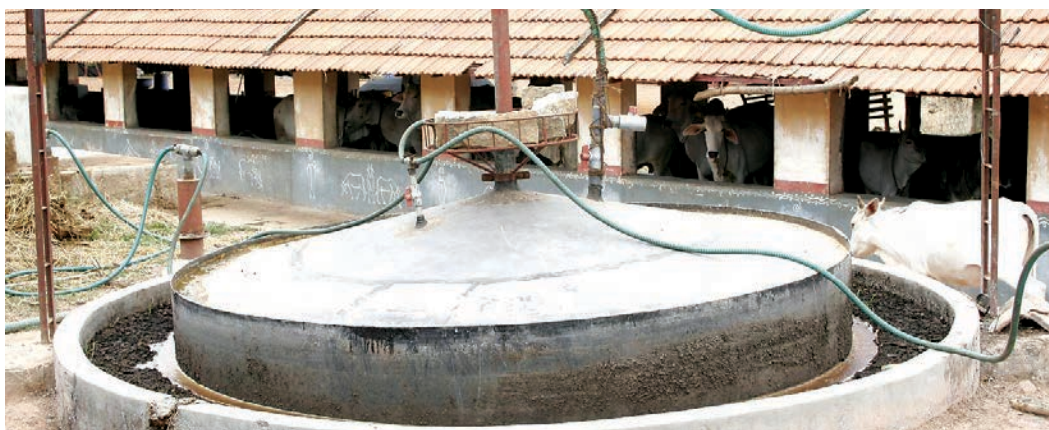
Fig.3.11-Biogas (Gobar gas) plant
