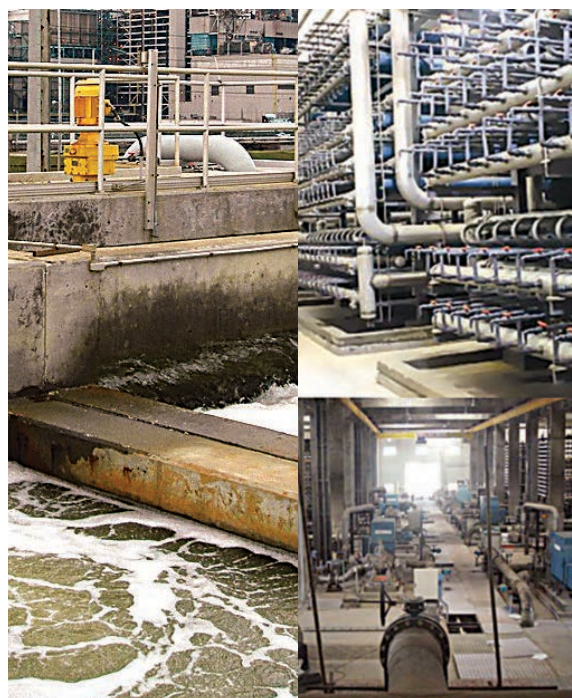
Fig. 2.12. The Desalination Plant at Minjur, Thiruvallur Dt.,
