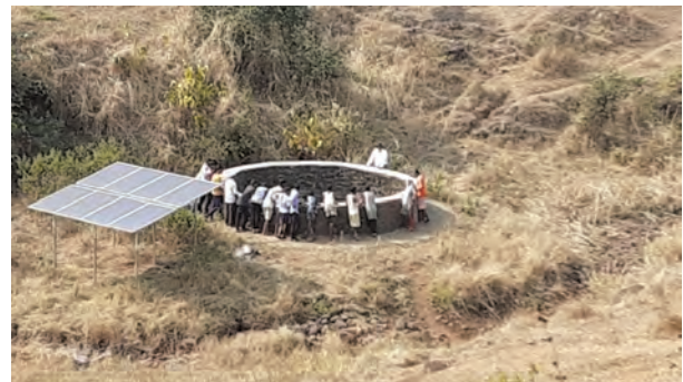
Construction of well through public participation
