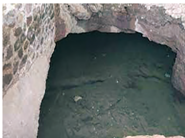
Water Devtake at Sinhagad, District Pune
