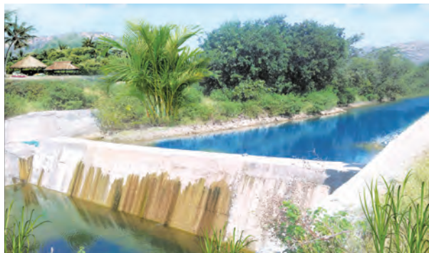
Nala Bunding –cement nala bunding
